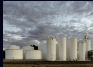
Tank storage facilities
